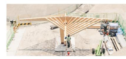
Glulam is also one-tenth the weight of steel and onesixth the weight of concrete; which allows for shorter installation time, lower installation cost and a faster return on investment. Mass timber products, such as glulam, that use raw materials from sustainably managed forests, provide an effective decarbonization solution to the built environment.
