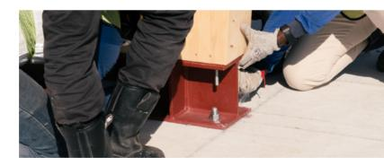
Both lead to more standardized and efficient assembly, translating to overall savings on building construction cost. The bolted modular supports significantly reduce carbon steel usage, enabling carbon footprint reduction, and reuse for future modifications.
